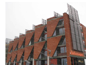
Roof mounted solar thermal collectors feeding the wider DH network in Western Harbour in Malmo, Sweden
