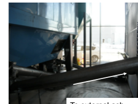
To external ash collection bunker
