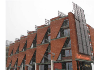
Roof mounted solar thermal collectors feeding the wider DH network in Western Harbour in Malmo, Sweden
