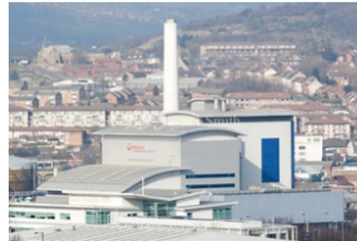
Sheffield city wide DH scheme fired with heat from waste incineration Copyright © Trevor Smith
