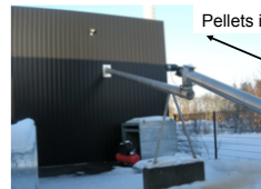
From silo into boiler
