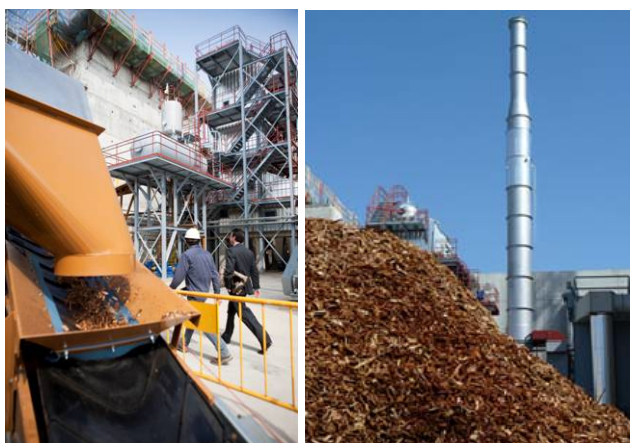
Figure 13: Actual picture of the Biomass plant
