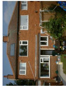
Roof integrated flat plate solar thermal collector for DHW generation
