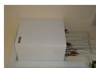
(left) Heat exchanger for hot water and space heating provision for a flat connected to DH
