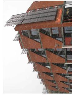
Roof mounted solar thermal collectors feeding the wider DH network in Western Harbour in Malmö, Sweden
