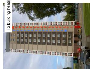
A block of flats using a central boiler to feed a distribution system is compatible for connection to a DH heating scheme provided that operating temperatures are suitable
