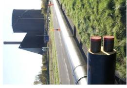
Work undertaken under the International Energy Agency and BRE suggested that heat distribution losses can be reduced by 20-37% in twin pipe systems relative to single pipe systems
