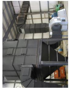
Multi cyclone dedusters provide the removal of ash from the flue gas to prevent PM emissions.
